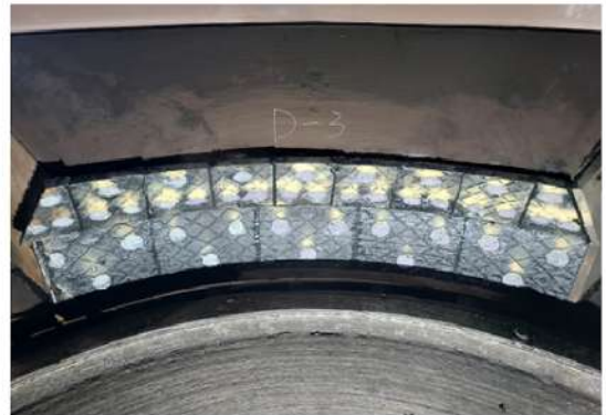
4. Deflector Liner 조립완료
