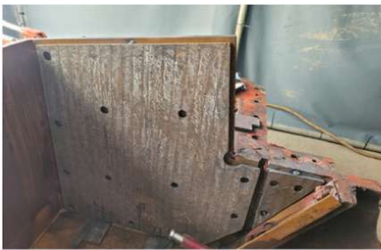
5. Opening Cover 초경 Liner 취부
