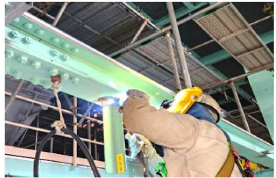
2. #1 "A" CASING SUPPORT WELDING
