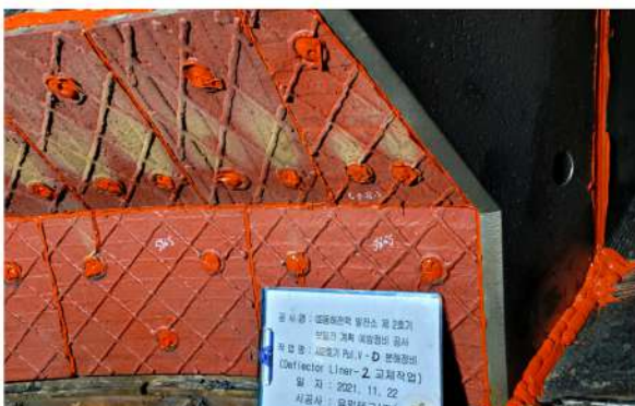
7. Deflector Liner 부착
