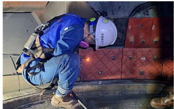
6. Deflector Liner 취부작업
