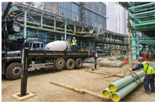
5. #2 "A" CASING CIA PIPE 운반
