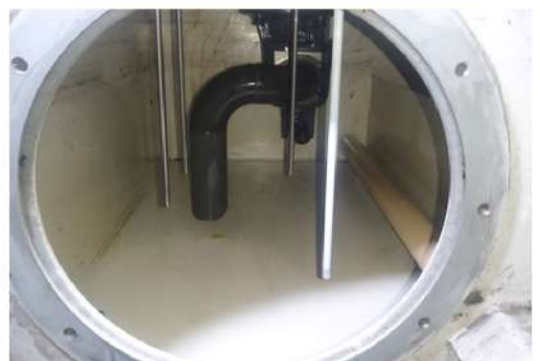
8. LUBE Oil Tank Cleaning
