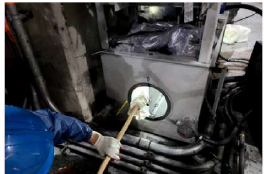
6. HPU Oil Tank Cleaning
