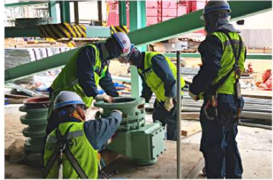
2. #1 "A" CASING AIRLOCK FEEDER 설치
