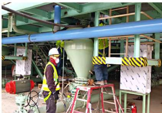
7. #1 "A" CASING SUPPORT 설치
