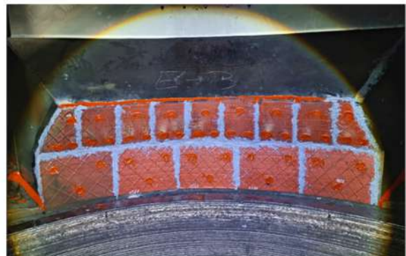
8. Deflector Liner 교체완료
