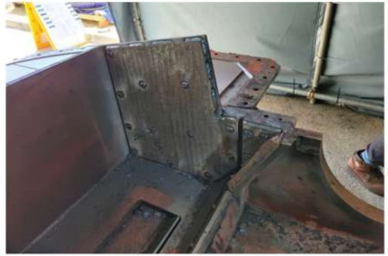
4. Opening Cover 용접 후
