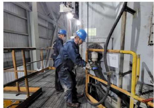
6. Seal Air Liner 조립
