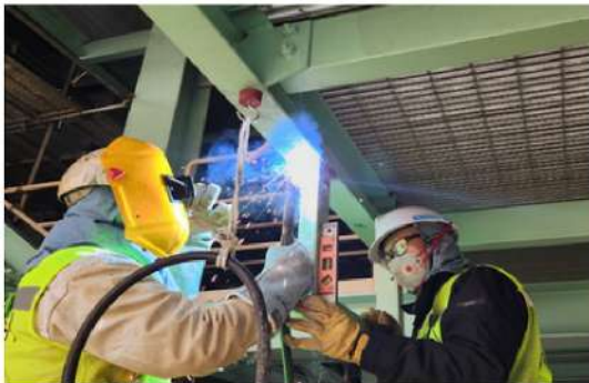
5. #1 "B" CASING SUPPORT 설치
