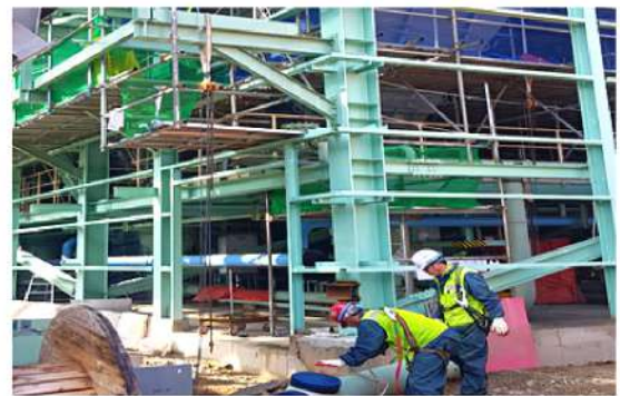
6. #1 "B" CASING PIPE RACK 배관 운반
