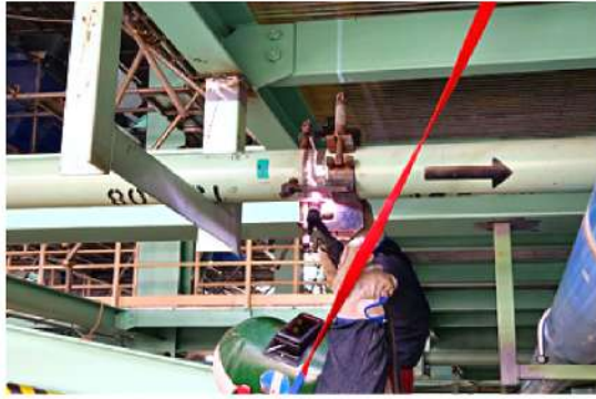
1. #1 "A" CASING FLUIDIZING 배관 WELDING
