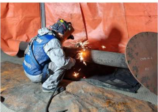
7. Burner Nozzle 육성용접
