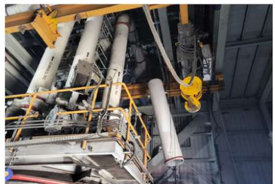
8. Coal Pipe 교체
