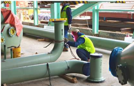
3. #1 "A" CASING TR BLOWER PIPE WELDING
