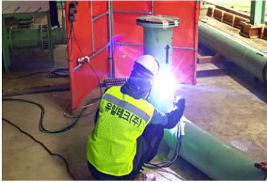
1. "B" Casing TR blower Pipe Welding
