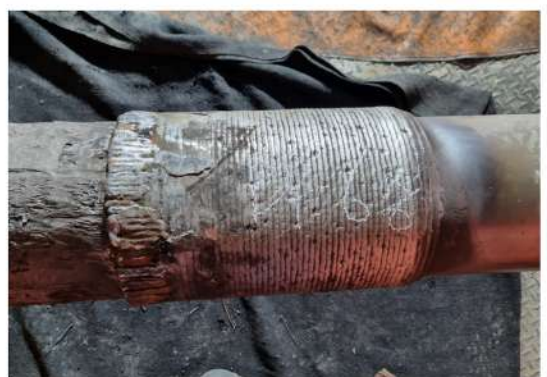
8. Burner Nozzle 육성용접
