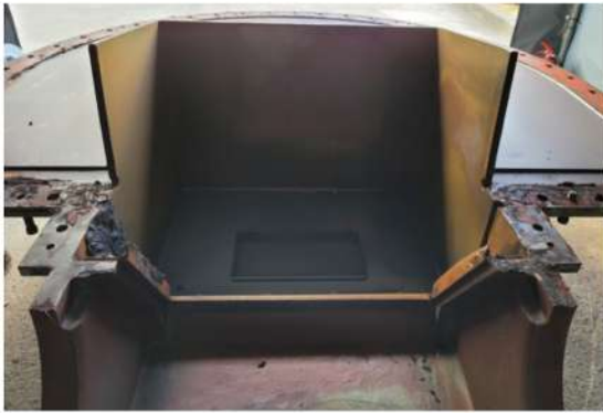
3. Opening Cover 용접 전
