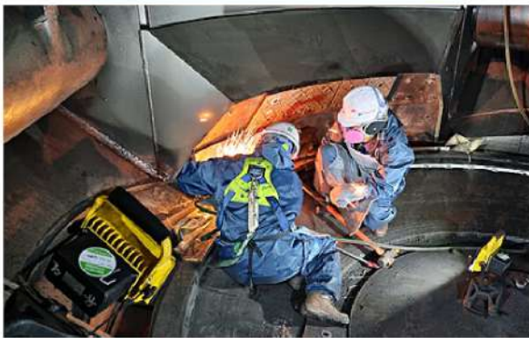
3. Deflector Liner 취외작업
