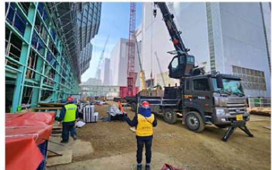
6. #1 "A" CASING AIRLOCK FEEDER 운반
