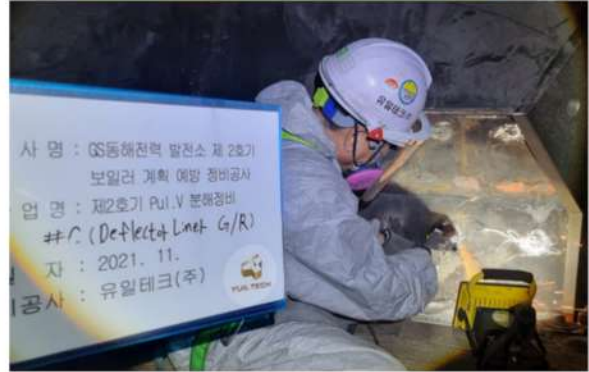
4. Deflector Liner 취외작업
