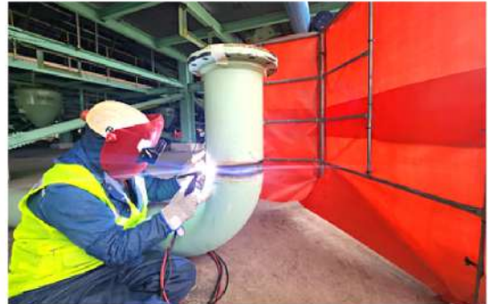
4. #1 "A" CASING TR BLOWER PIPE WELDING
